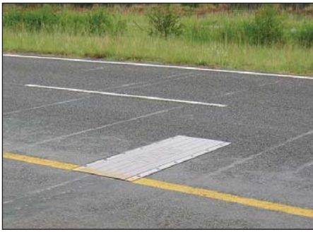
Figure 1 Typical half-lane high-speed WIM installed on a freeway. Another sensor and a set of inductive loops are across the median, for the other direction of travel
