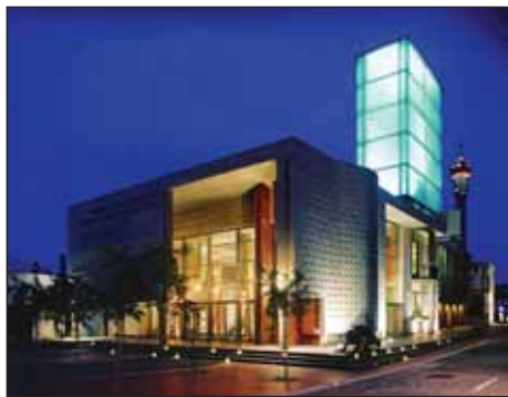
Concrete has been used with great skill in the Constitutional Court
