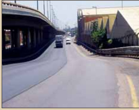
SMA surfacing on fast and middle lanes
