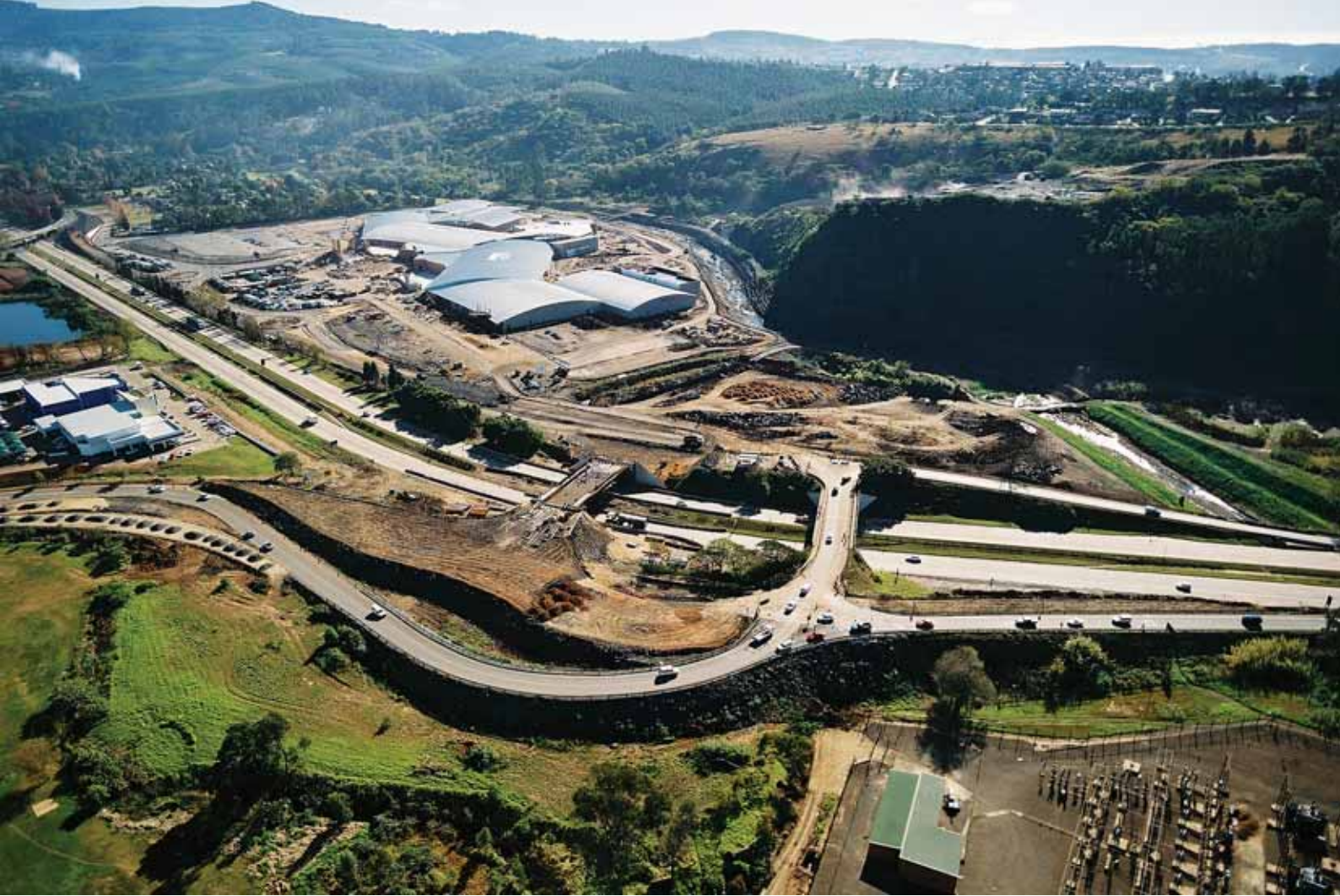
Left: Rotary Interchange at Liberty Midlands Mall; above: Construction in progress
