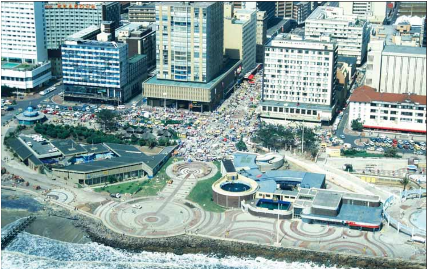
In an extensive urban-design project on the Durban beachfront, through traffic was diverted inland and landscaped parking introduced
