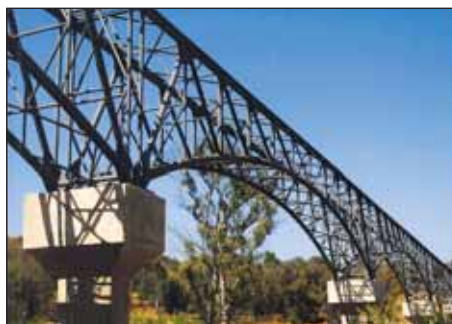
Leeuwkop Relief Outfalls sewer pipe bridge
