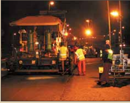
Paving the asphalt base at night
