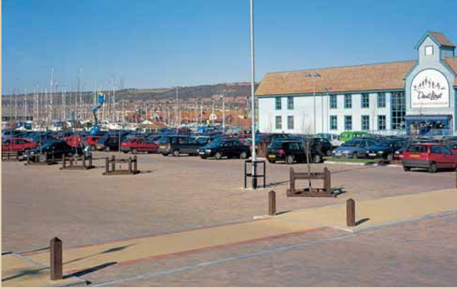
An example of Formpave storm water control system at a recently constructed leisure centre (sporting complex) in Port Solent, England. The car park is situated over a sub-base reservoir system which is used to store rain water absorbed by the paved surface
