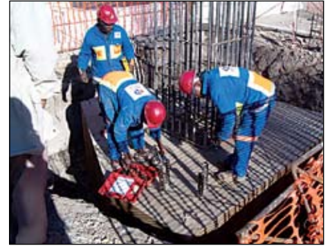
Figure 5 Preparation of CHSL testing
