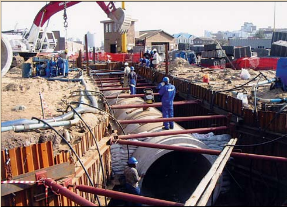
Concrete piping was chosen for this stormwater relocation project in Durban. The picture shows a section of a 2,5 diameter concrete pipe being bedded into position. Each pipe section weighed 13 t and included half a ton of steel
