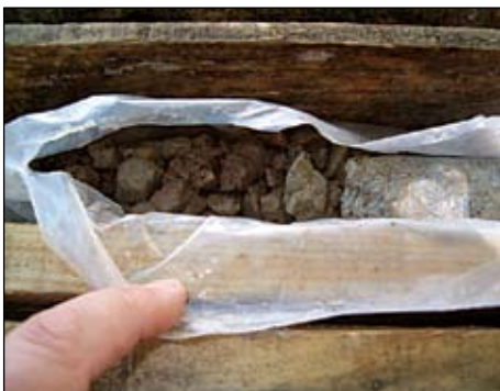
Figure 7 Contact between pile concrete and base
