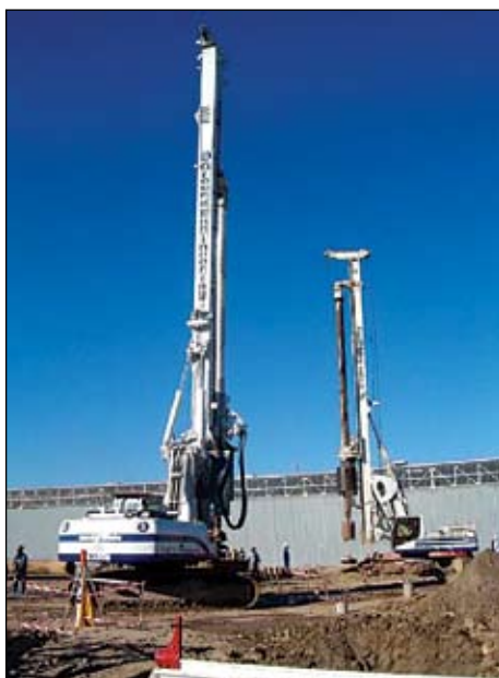
Figure 2 Casagrande and Soilmec auger rigs
