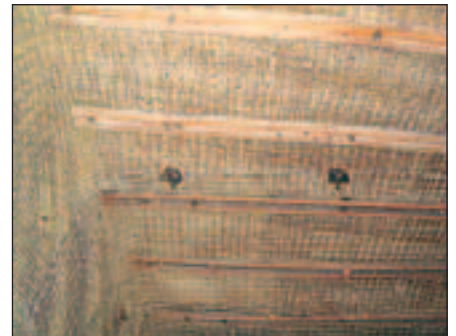
Rock support during and after installation
