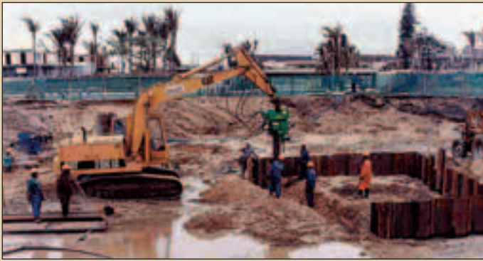
Installing sheetpile cofferdam for deep liftshaft pit (Durban Point area)
