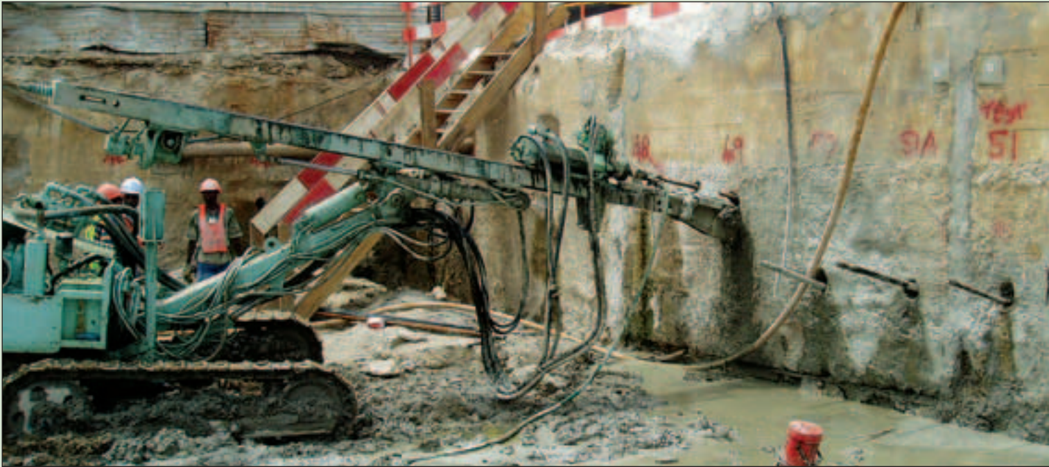
Geofranki installing the Franki-Titan anchors through the diaphragm wall
