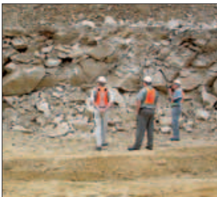
Extensive damage to sandstone rock after pre-split and bulk blasting
