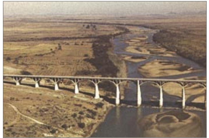
Looking downstream: the new Bethulie road and rail bridge across the future dam basin
