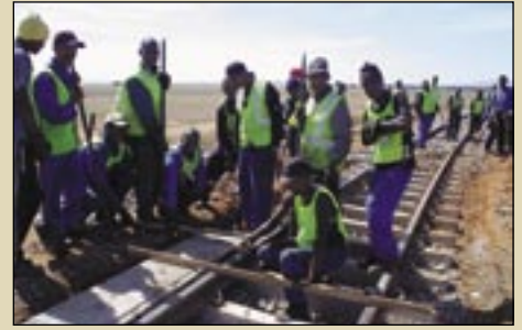
Kalbaskraal: Placing of cross blocks
