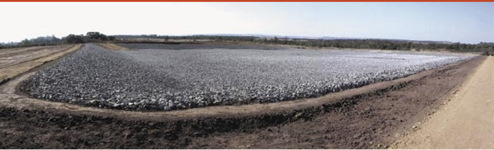
Completed construction of the first 2,5 ha capacity waste cell
