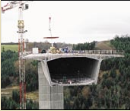
Work in progress on the Sioule Viaduct
