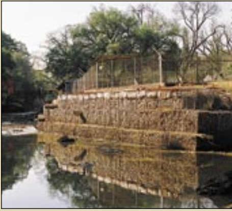
The Apies River – after its banks were stabilised
