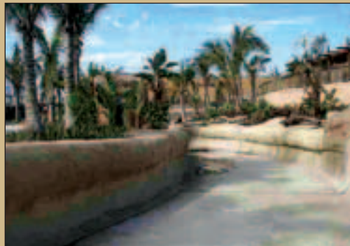
Caption: Canals under construction at uShaka Marine World
