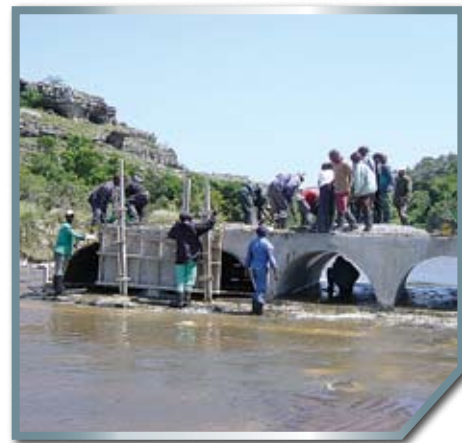
► Causeway construction in progress showing semi-skilled labourers at work
