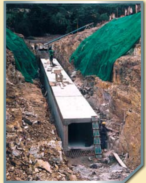
► Eighty per cent of East London's water is treated at the Umzoniana water treatment works, which uses the Umzoniana dam as a balancing dam. The raw water to the dam is obtained from the Buffalo River via five high-lift pumping mains, three of which discharge into surge chambers 128 m above the level of the river at the head of two 900 mm diameter gravity mains. These gravity mains discharge into the inlet portal of a 200 m long tunnel. After passing under a low ridge the tunnel discharges into the dam. Owing to the critical nature of the raw water supply system, the whole supply system is duplicated, except for the tunnel. After the collapse of the centre sections of the
