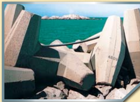
► Dolosse effectively strengthening the breakwater at Coega
