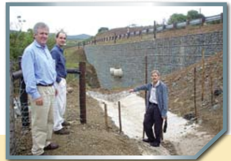
► Mike Deeks, Johann du Preez (2005 treasurer, Amatola Branch) and Dawie Botha on the Kei Mouth road near the turn-off to Magrangeni – an example of a reinforced earth wall where galvanised welded mesh was used, faced with carefully placed rock and obtaining its strength from the tie-back strips that are embedded in the backfill
