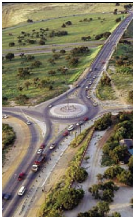
Traffic circles on the Hans Strijdom Interchange
