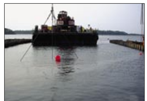
Installation carried out by means of cranes and barge
