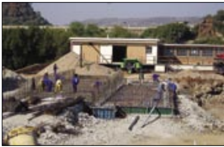
Bospoort Dam: Structural concrete commences for the GAC filters
