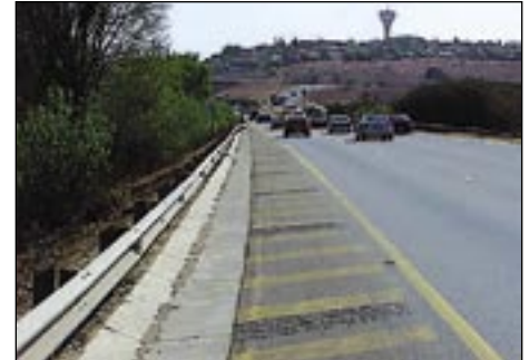
Details at structures
