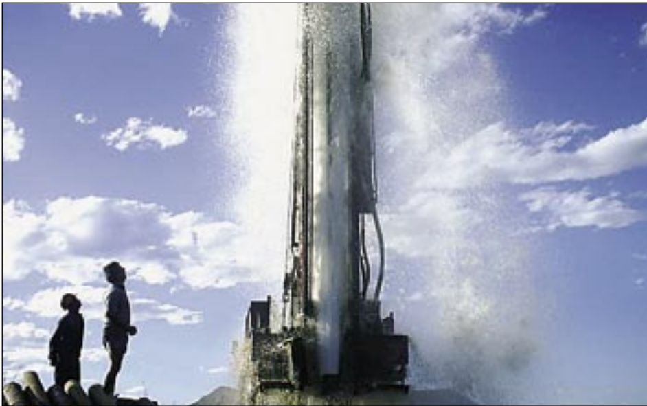
Taken during drilling: water is lifted from the borehole using compressed air to give a first estimate on the yield of the borehole
