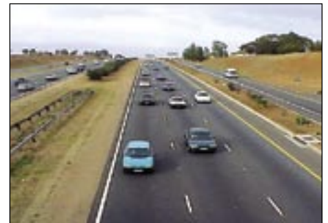
Upgraded road section
