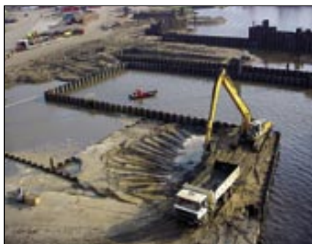
Dredging an installation of the steel sheet piles
