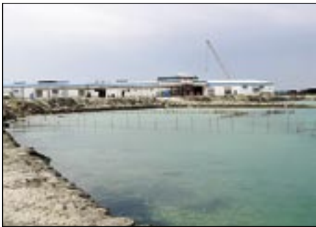
Al-Ezzel site of intake structure at high tide
