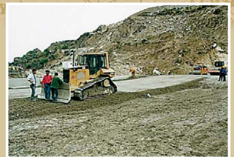
Coffer dam construction
