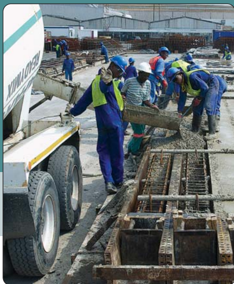
Pouring concrete into precast pile moulds
