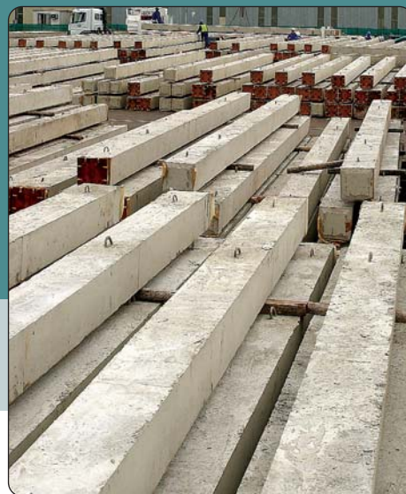
Precast pile storage yard
