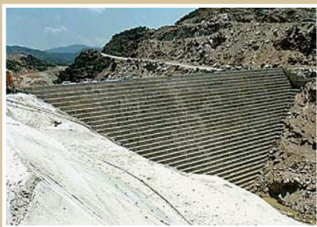
Completed coffer dam
