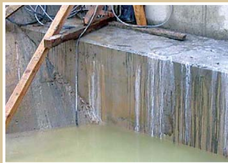
GE-RCC facing finish
