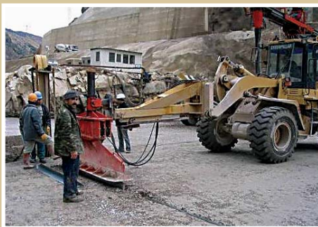
Joint forming in compacted RCC
