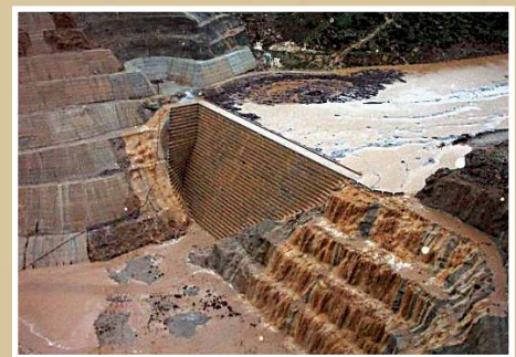
Coffer dam during severe flooding (January 2004)
