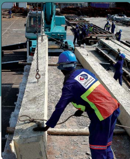
Loading precast piles for transport
