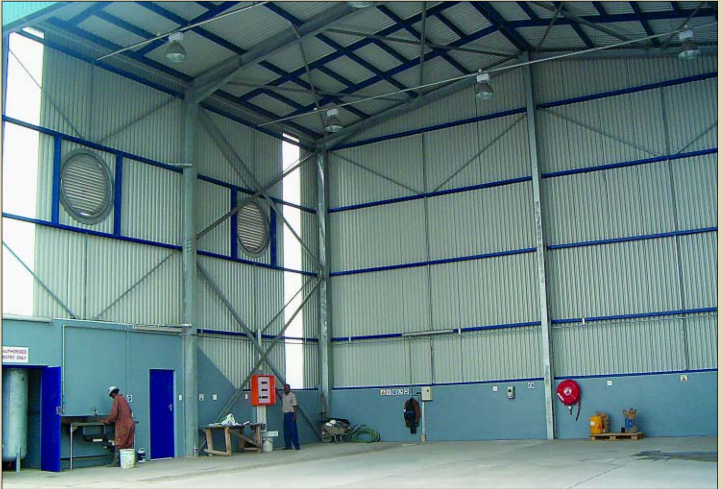
Interior of the MHA workshop of SAPO provided by Protekon at Maydon Wharf, Durban Port
