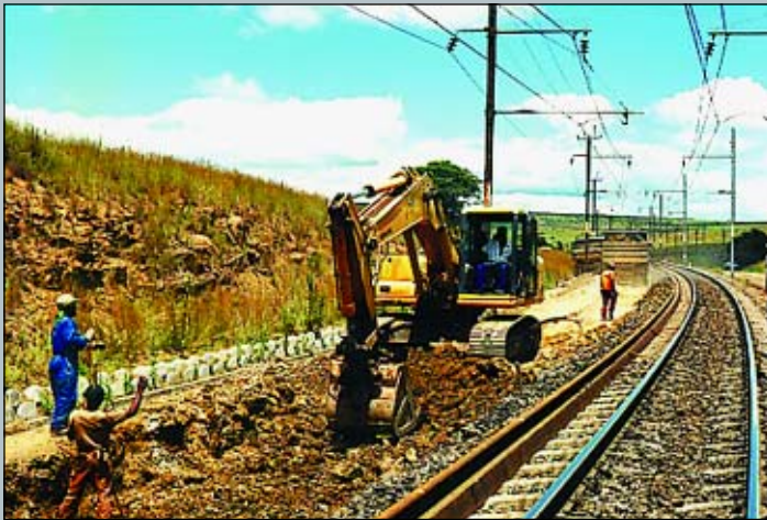
Figure 1 Formation rehabilitation on the Broodsniersplaas - Richards Bay coal line
