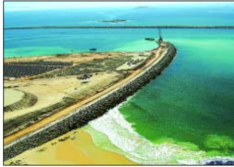
The western breakwater viewed from the landside
