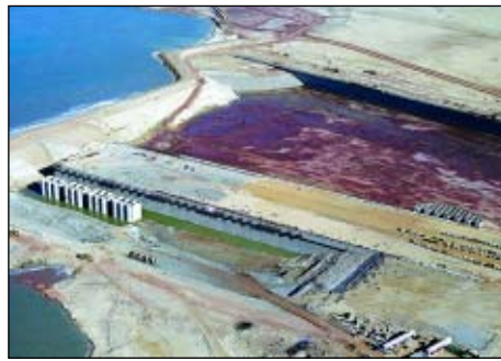
The dry excavation prior to flooding of the basin
