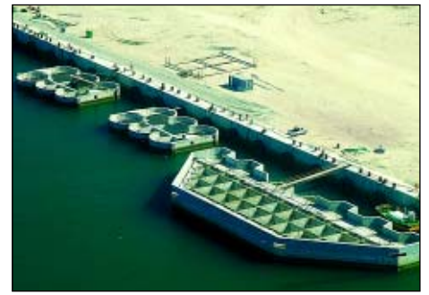
The western and eastern breakwater head caissons prior to float-out
