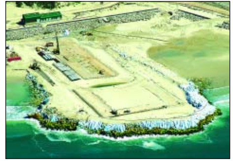
The sand bypass temporary works under construction
