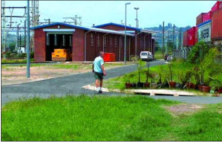
The new building at Umbilo that houses the under-floor wheel lathe. Site agent Ricky du Plessis is crossing into the new access road
