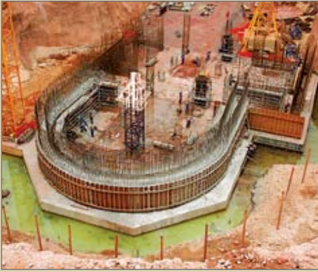
View of the primary crusher base under construction
