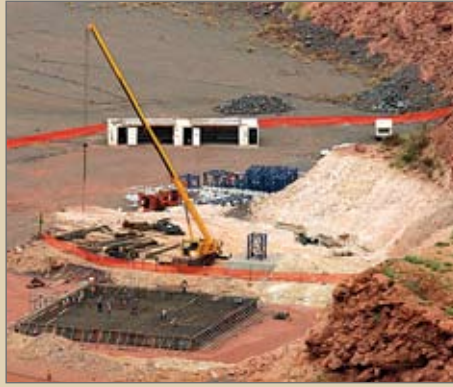
Construction of the secondary crusher base
