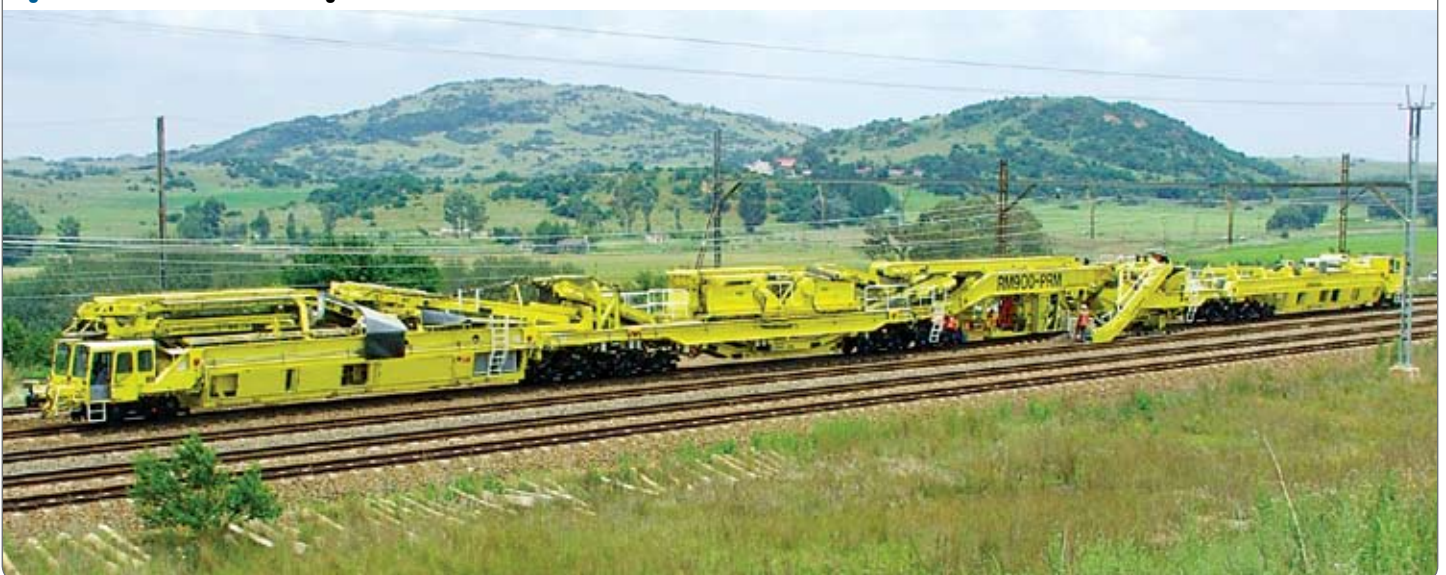
Figure 7 The RM900 ballast cleaning machine
