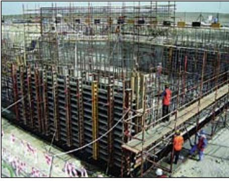
Construction in progress: Al-Ezzel Power Station, Bahrain
