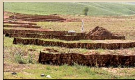
The start of the Izinga Ridge erosion control project in November 2004
