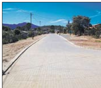
Lang Street after
