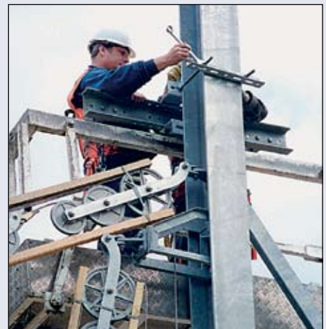
► Top: Figure 3 Operating revenues for social infrastructure projects such as hospitals are subject to less risk (courtesy NHS Estates) ► Bottom: Figure 4 Railway equipment is expensive to replace (courtesy CTRL)
