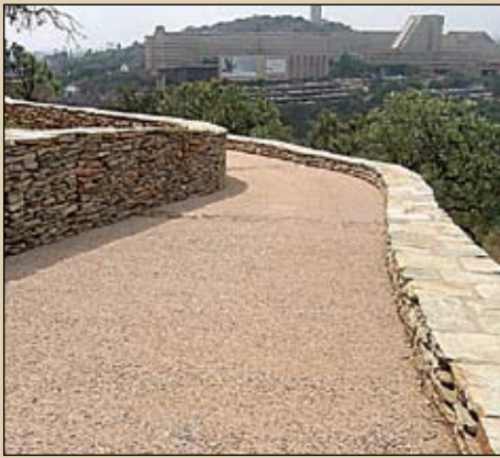
Freedom Park, where exposed aggregate finishes played an important part in the award-winning landscaping
