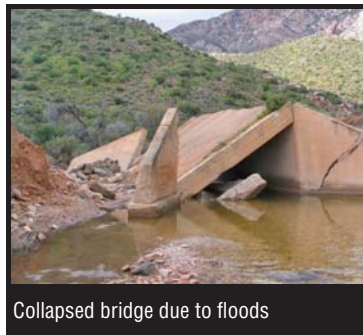
Blocked stormwater drain destroyed
