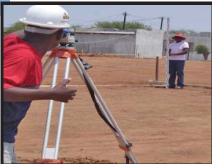
Elvis surveying after backfilling foundation complete for the civic hall
