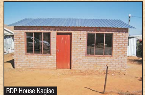
Construction of RDP House
