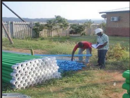
Counting of pipes for water project and Civic centre
