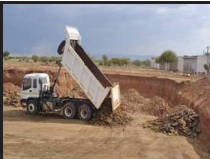
Dump truck offloading selected fill
