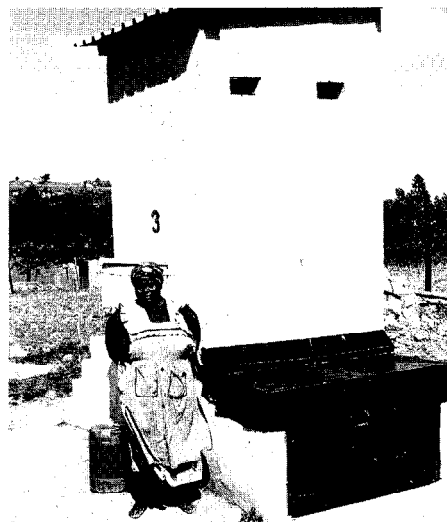
Figure 3 Completed urine diversion toilet unit at Sinyondweni
